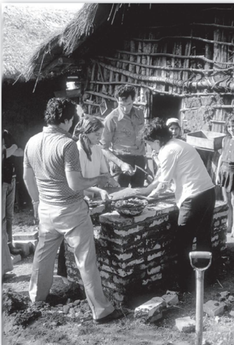
Building a fogón. A new kitchen will be constructed around it.
